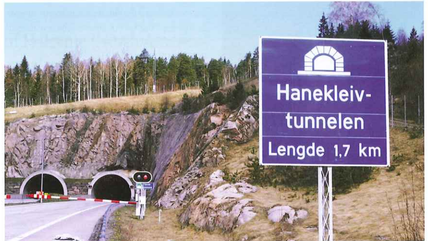
The Hanekleiv Tunnel in Vestfold, Norway, runs through highly unstable rock conditions and was opened to traffic in October 2001
